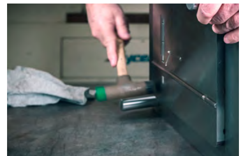
Installing the insert
